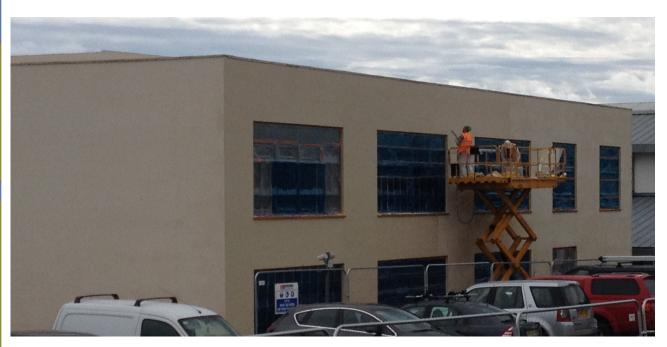
The rear and sides walls of the Sixth Form Centre are coated with the weather-proof render and are now close to completion.
